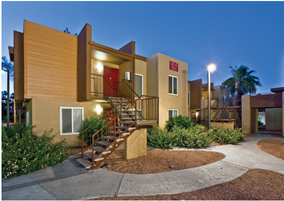
SCOTTSDALE GATEWAY — TEMPE, ARIZONA
